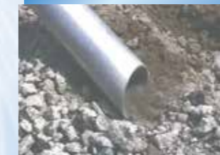
▲ Debris and rubble
